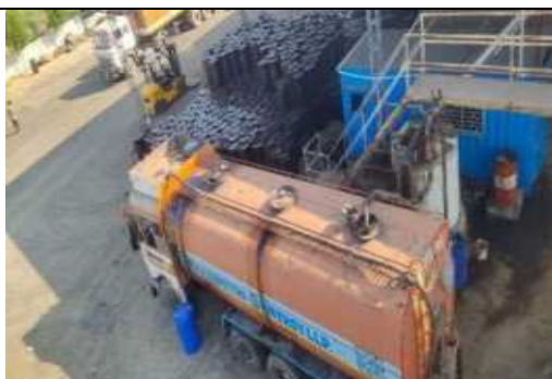
Emulsion Bitumen Loading Point
